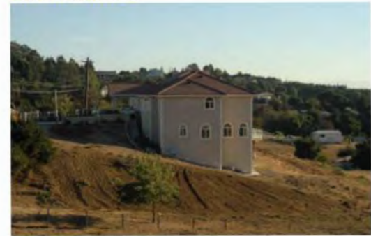
This single-family home does not step down the hillside, resulting in a tall downslope wall that is highly visible and out of scale with surrounding neighborhoods. (Guideline B-4)
